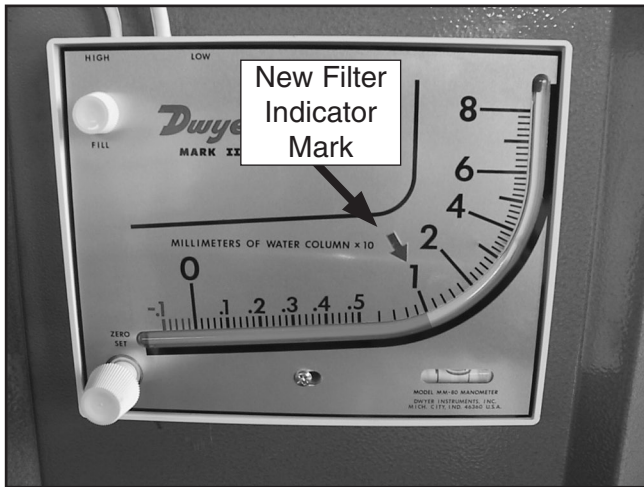
Figure 28. New filter installation mark example.
