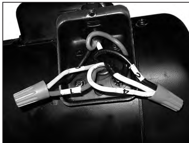
Figure 62. 110V motor wiring.
